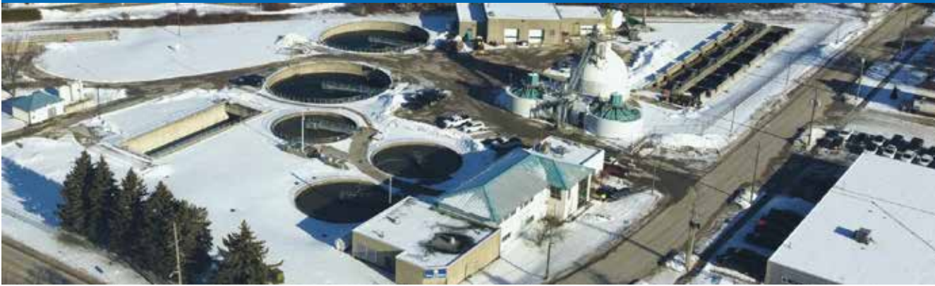
Midland's water treatment plant. Source: Town of Midland Water and Sewer Services tinyurl.com/v4r62hre
